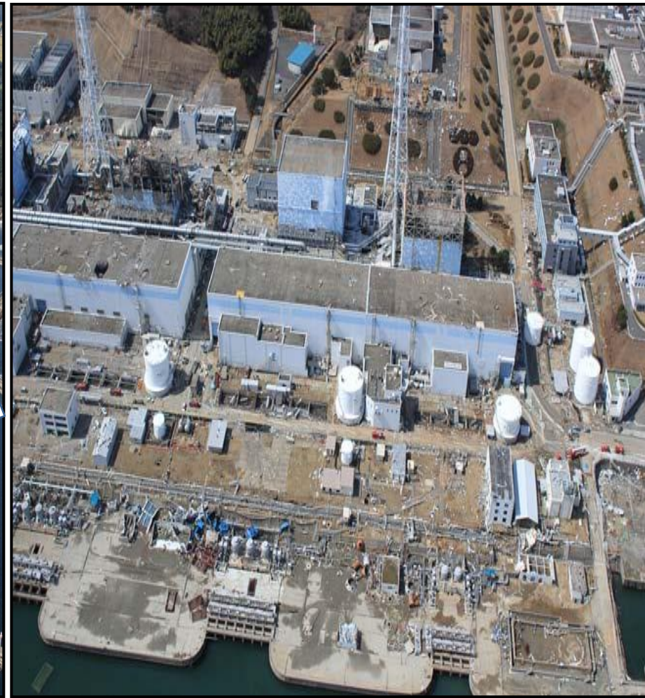
After the Earthquake and Tsunamis
